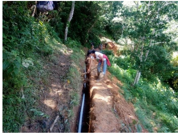
Progress of trenching and laying pipe for new transmission main
