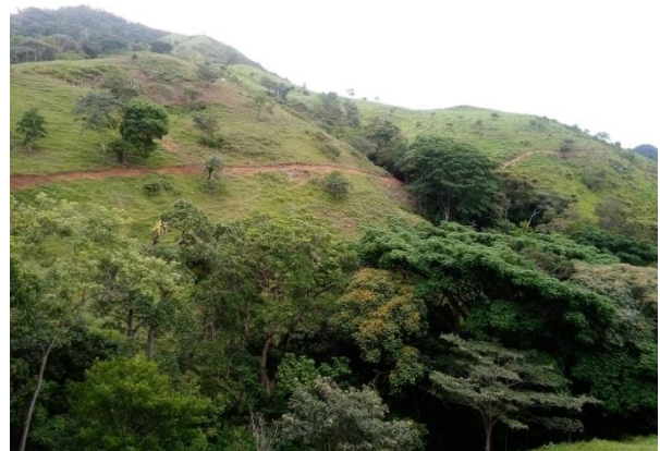
Trenched pipe route going from a new source to the storage tank
